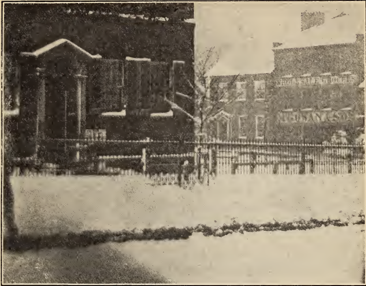
WILLIAM R. DICKINSON RESIDENCE, CENTRAL BUILDING.
